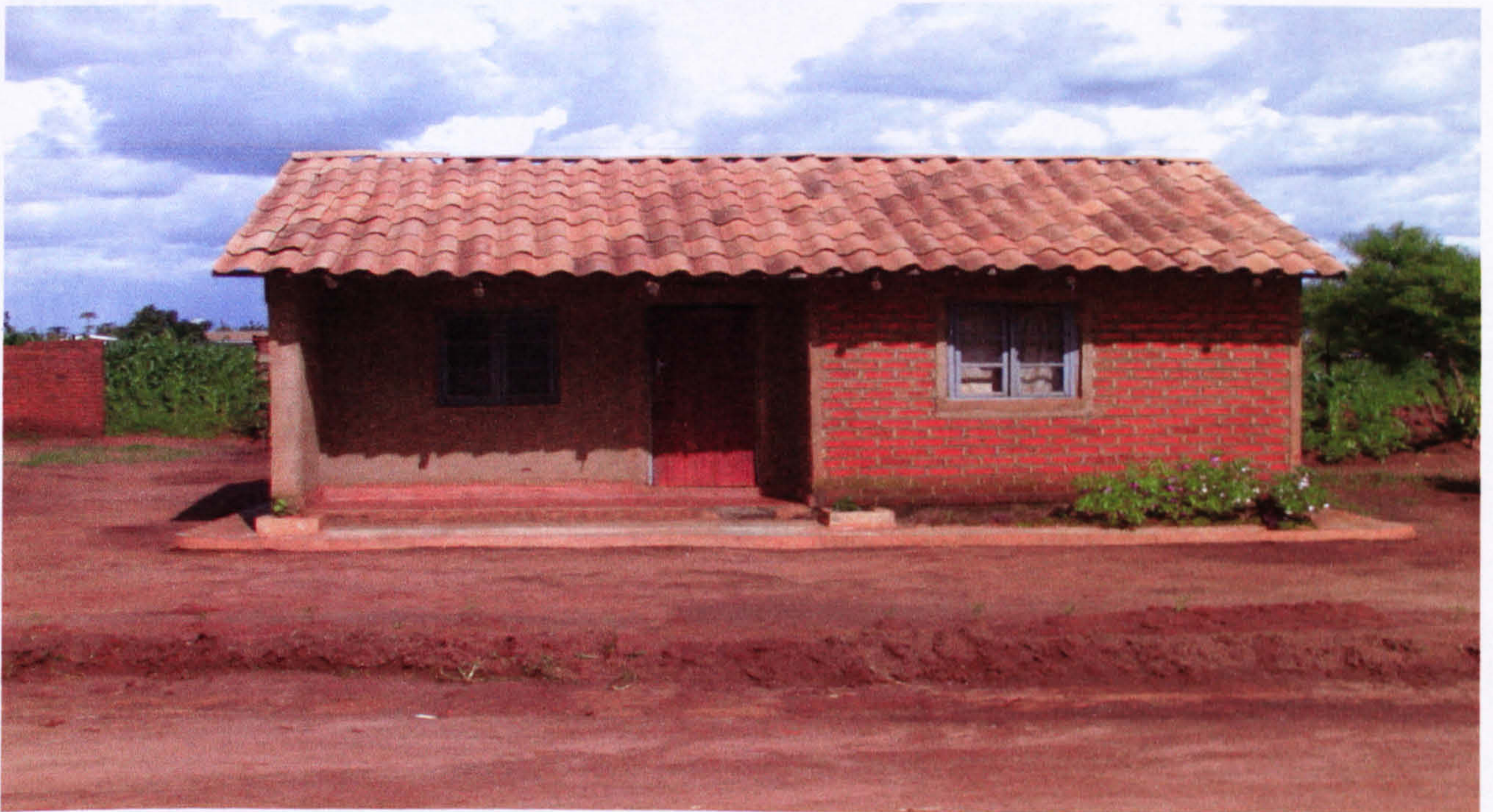
Plate 5.5 Another intermediate technology house. Although the windows have been improved, the walls are not fully protected from the strong irradiance during the late morning and early afternoon. Note the insolation through the window and the exposure of half of the front wall. Note the small verandah and plinth.
