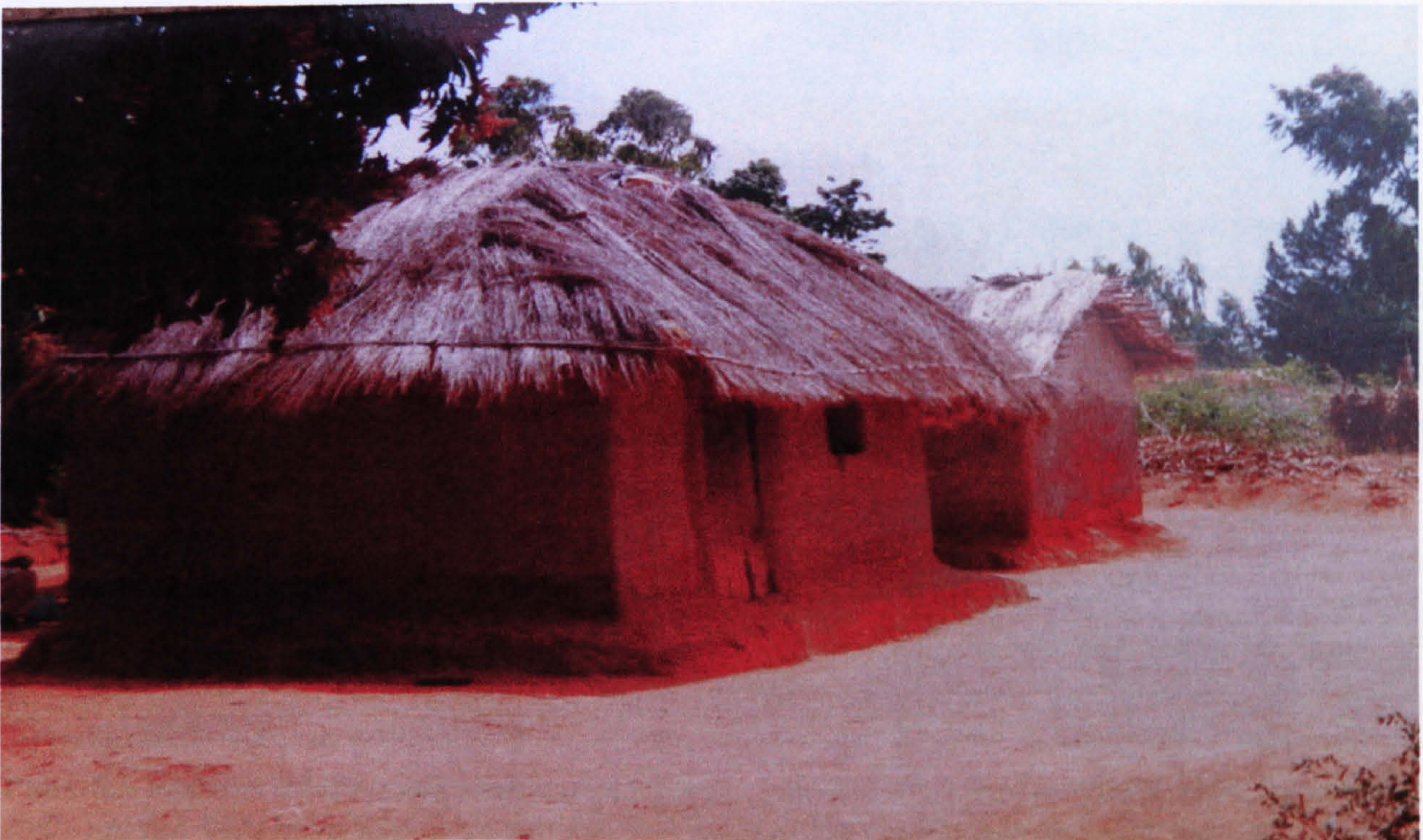
Plate 5.3 The same traditional house taken at a different hour of the day to illustrate how the roof protects all the walls from the strong irradiance at the high hour angles.
