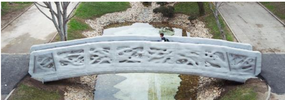
Figure 12 The first printed concrete pedestrian bridge by using binder jetting technique. Located in the urban park of Castilla-La Mancha in Alcobendas, Madrid (Markopoulou,Rodrigo Aguirre et al. 2016). .
