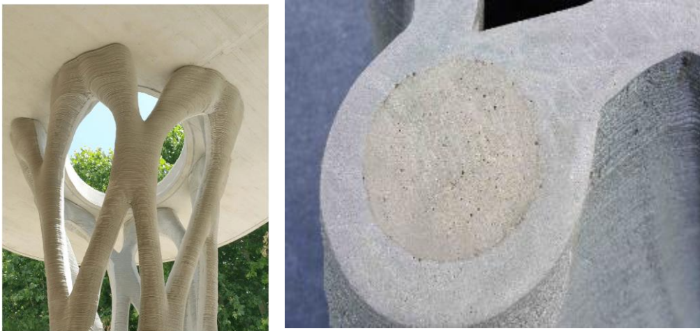
Figure 20 XtreeE pillar in Aix-en-Provence, built in France 2016 (left) and section of the pillar (right) (Gaudillière et al., 2019).
