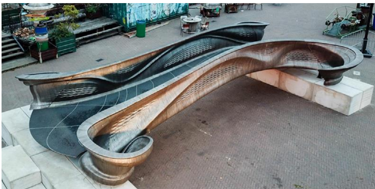
Figure 14 The MX3D bridge (Tim Geurtjens, 2015).
